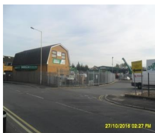
Resin Plant & Barrel Farm Now~ Emerson Cranes
