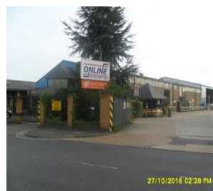
Loc.400 & No 2 Car Park Now~ OnLine Roadways
